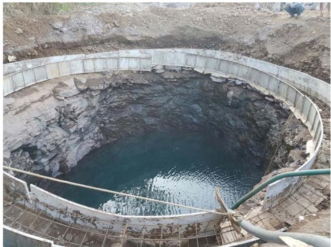
**Early stages of well construction where the ground was saturated with water.**
